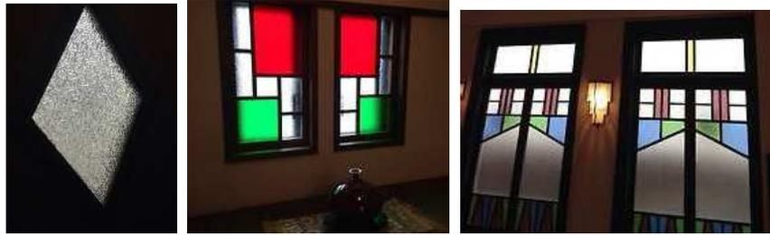
Figured rolled-plate glass, original colored glass (red and green), modern colored glass.
