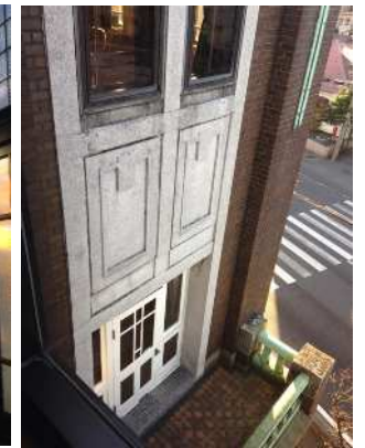
View of 2nd floor balcony from above.
